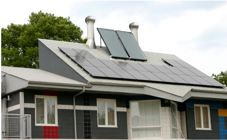
1. House with solar panels and wind turbine vents
