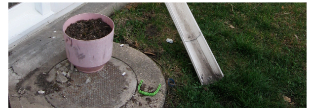
10. Rain gutter emptying into lawn
